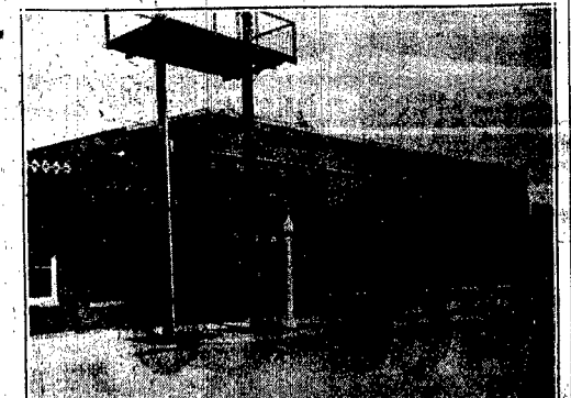
Constructed in 1928 at an estimated cost of $5000, Wayne's light plant supplies electricity to residents at a minimum rate.
